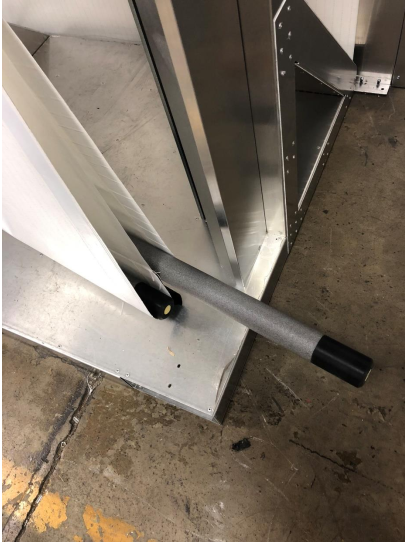
Figure 22: Removal of Tension Pipes
