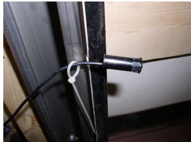
Remove Photo cell
