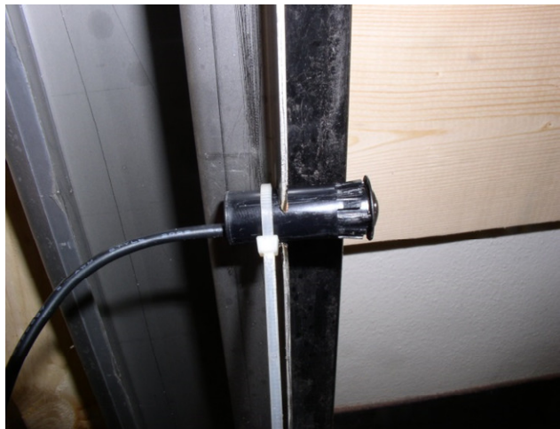
Push Photo cell through hole
