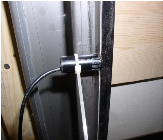
Install tie wrap snug around the barrel of Photo cell
