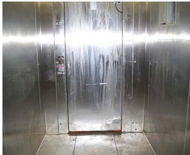
5'10" x 11'7" x 7'6" H Walk-In Freezer with Floor
