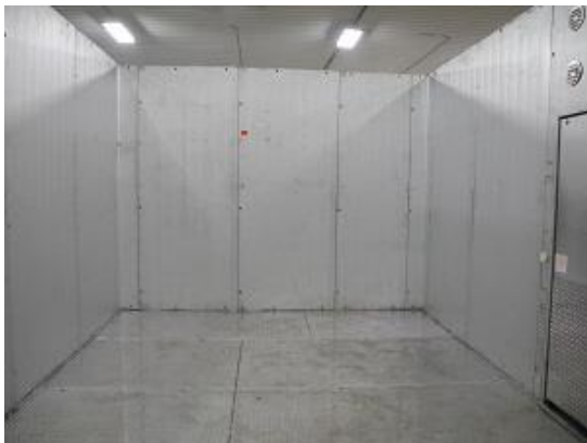
12'6" x 21'2" x 10' H Walk-In Freezer with Floor
