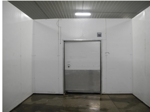
21' x 24' x 10' H Combination Walk-In Cooler / Freezer
