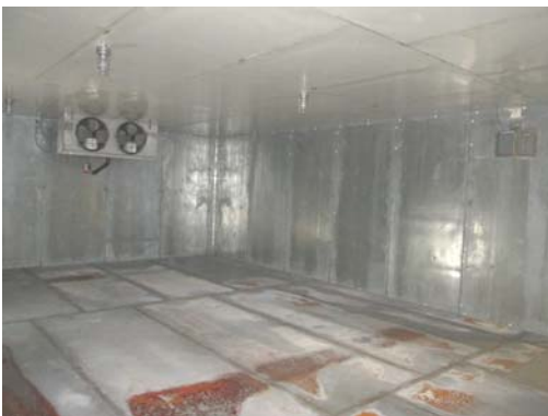
30'9" x 32'8" x 9'11" H Walk-In Freezer with Floor
