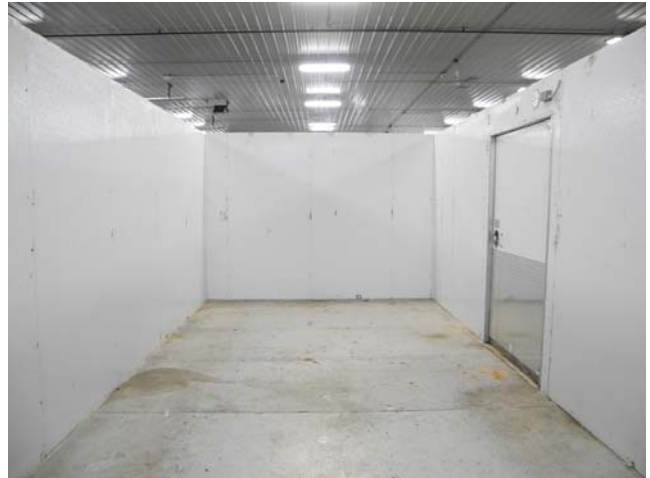
11'7" x 27'10" x 8'9" H Walk-In Freezer With Floor
