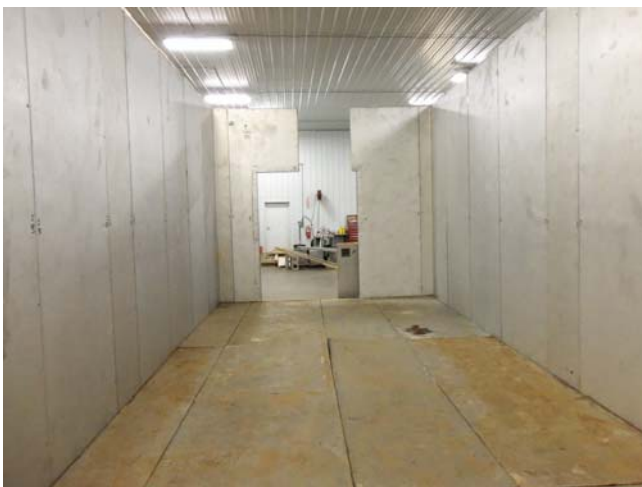
25'2" x 33'11" x 11'7" H Combination Walk-In Freezer With Floor
