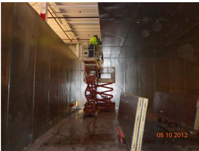
45'10" x 163' x 14' H Drive-In Cooler or Freezer
