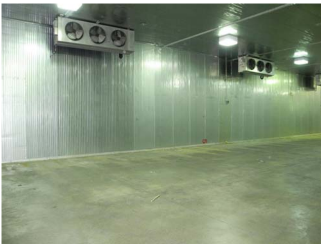
36'9" x 123'9" x 16'2" H Drive-In Cooler or Freezer
