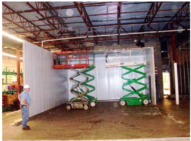
24'4" x 44' x 14' H Walk-In Cooler or Walk-In Freezer
