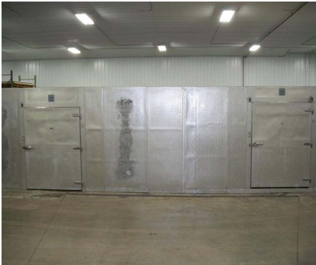
12' x 40' x 8'6" H Combination Walk-In Cooler/ Walk-In Freezer
